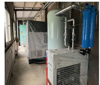
▲ Positioning and Alignment of Newly Installed Equipment
