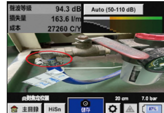
▲ Utilizing the LD500 to Locate Leakage Points and Quantify Leakage Volume
