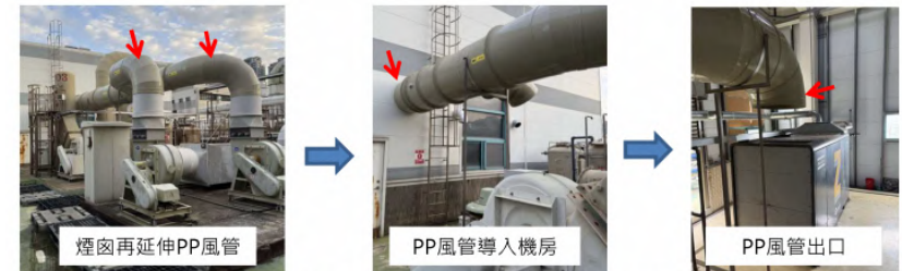
▲ Extending the general exhaust duct from the old plant to route into the CDA-8 room and blow directly toward the CDA-8 air intake
